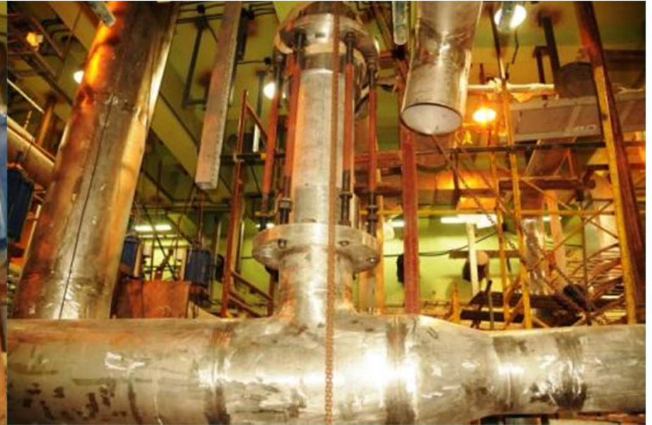
Sodium Piping Installation
