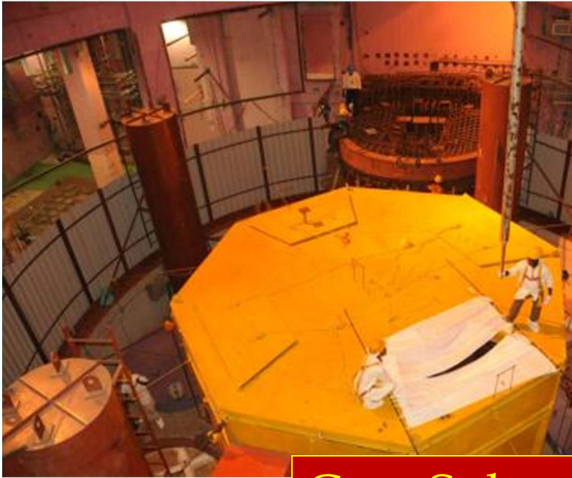
Core Sub assemblies erection
