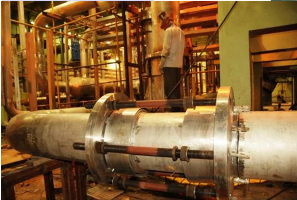
Sodium piping – Bellow fit up & welding
