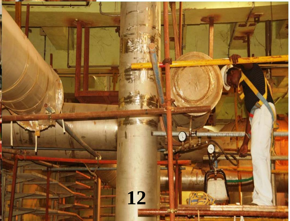
Sodium Piping Installation
